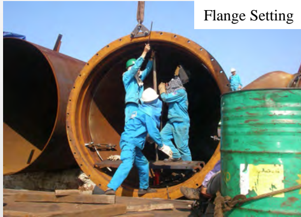
Intake Head assembly
