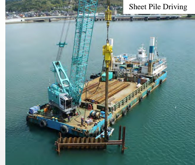
Sheet Pile Driving
