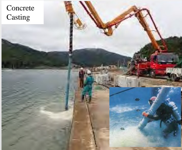
Revetment Construction
